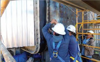
10' x 15' X 12" face-to-face fabric expansion joint belt and bolster replacement in a Louisiana gas turbine power plant
