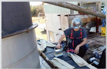
Gas turbine exhaust fabric expansion joint installed and spliced by Badger On-Site personnel
