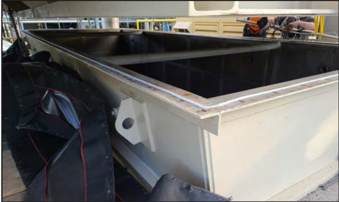
Badger's turnkey replacement service includes removing the existing fabric expansion joint, hardware assemblies, and backing bars
