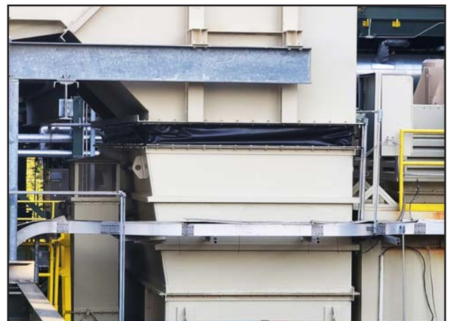
Badger's air inlet duct expansion joints eliminate the costly OEM zipper closure
